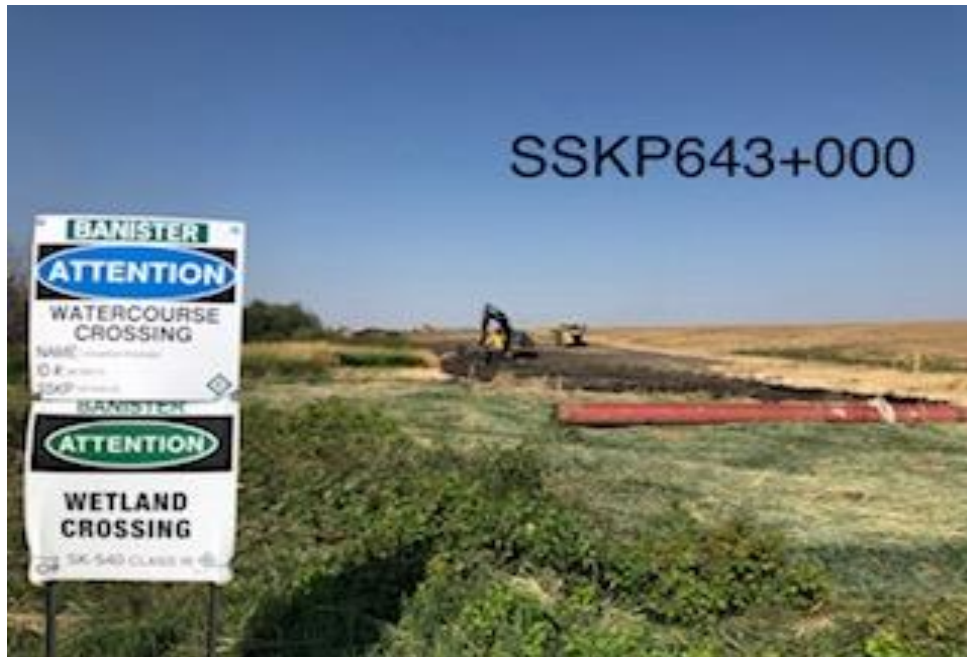
Ramp installation in a wet land crossing
