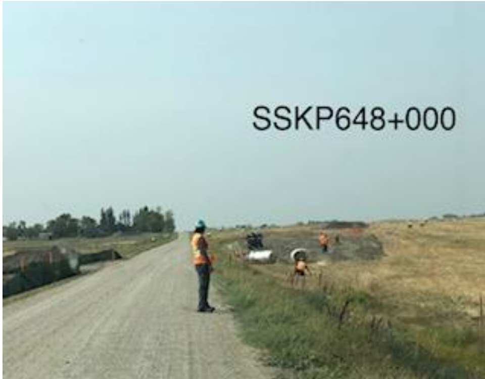
Stringing before ramp installation
